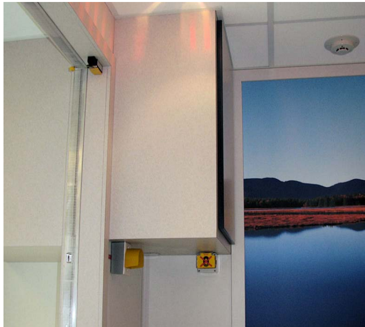
Guarded Magnet Quench Button in the Scan Room
