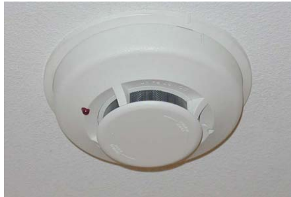
Figure 23: Smoke Detector
