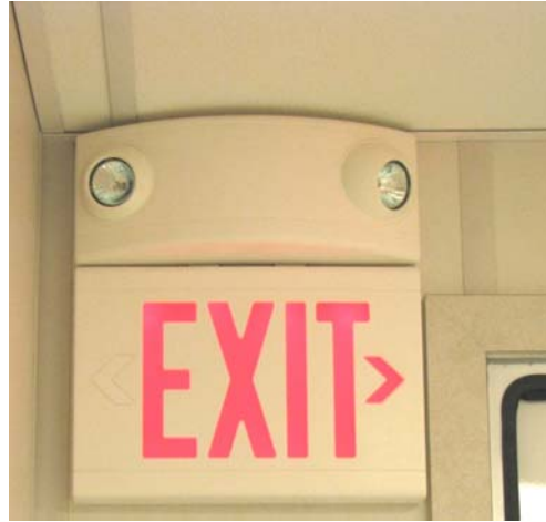
Figure 21: Emergency Lighting
