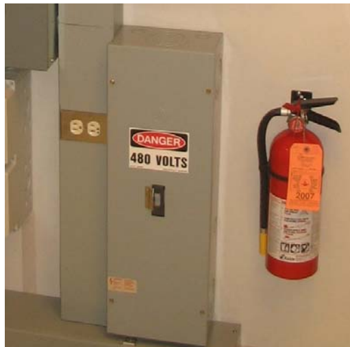
Figure 34: Shunt Trip
