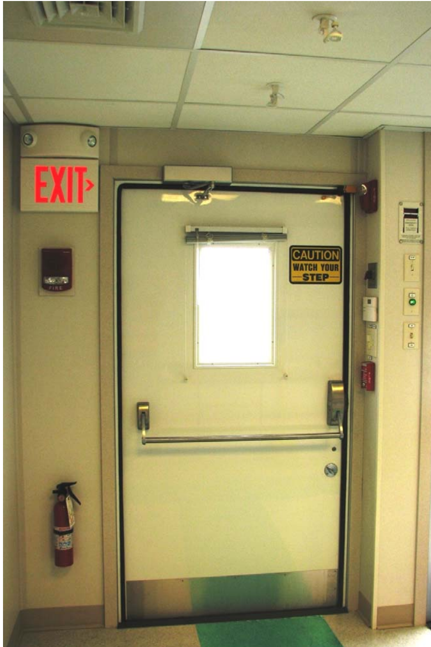
Figure 8: Exterior Staff Door
